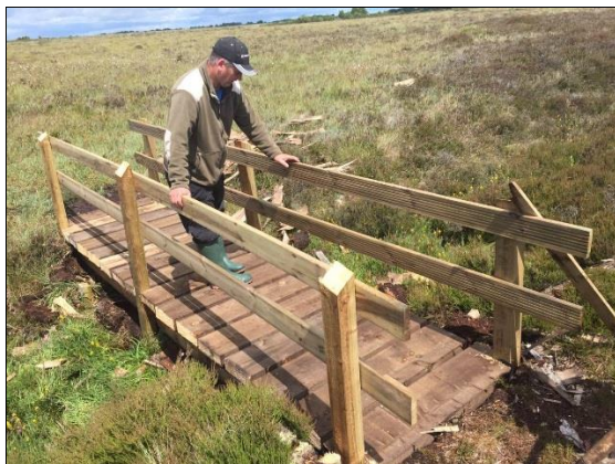
Access bridges built and maintained
