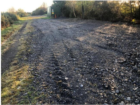
Parking and road access improved (2021)
