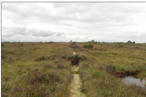
Bog restoration work (drain blocking)
